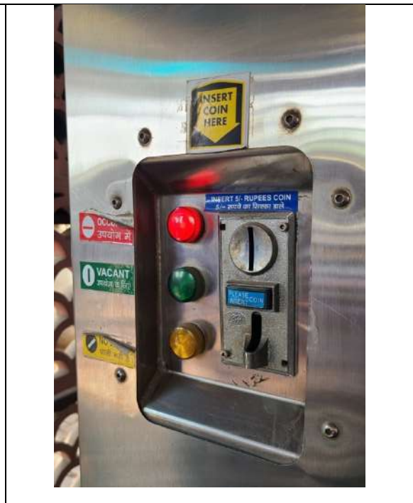
Automatic Smart Toilets System
