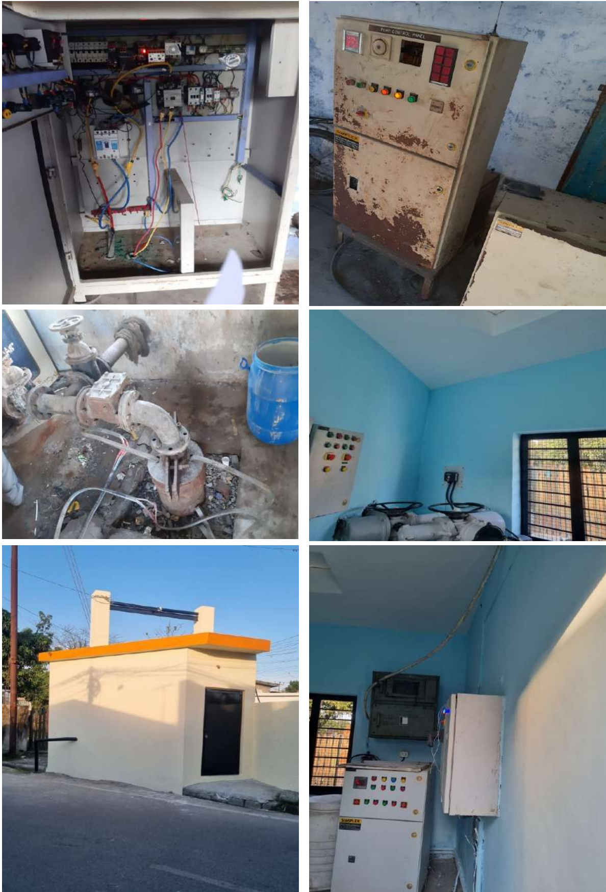
Figure 3: Implementation images from Dehradun Water Supply Project capital work
