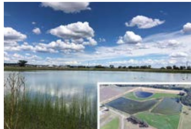
On this page, Top - Former Sewage Treatment Ponds Source: Parkes Champion Post, 2023 Middle - Water flowing into Parkes Wetland Source: Parkes Shire Council, 2023 Below - Current and former condition of the Wetland Source: Parkes Shire Council, 2023
