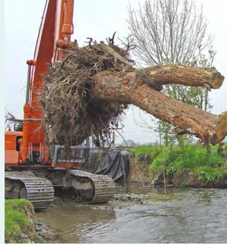
2. Moving root into position
