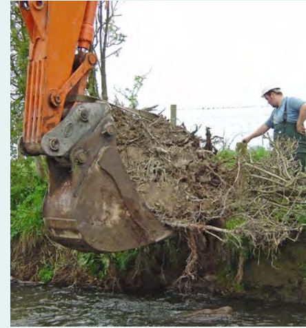
3. Installing Root Wad
