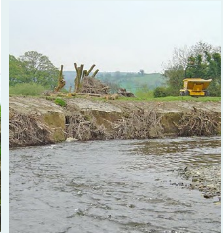
4. Right after installation
